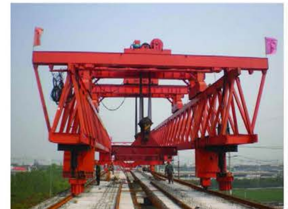
中铁一局施工现场 China railway first group construction site
