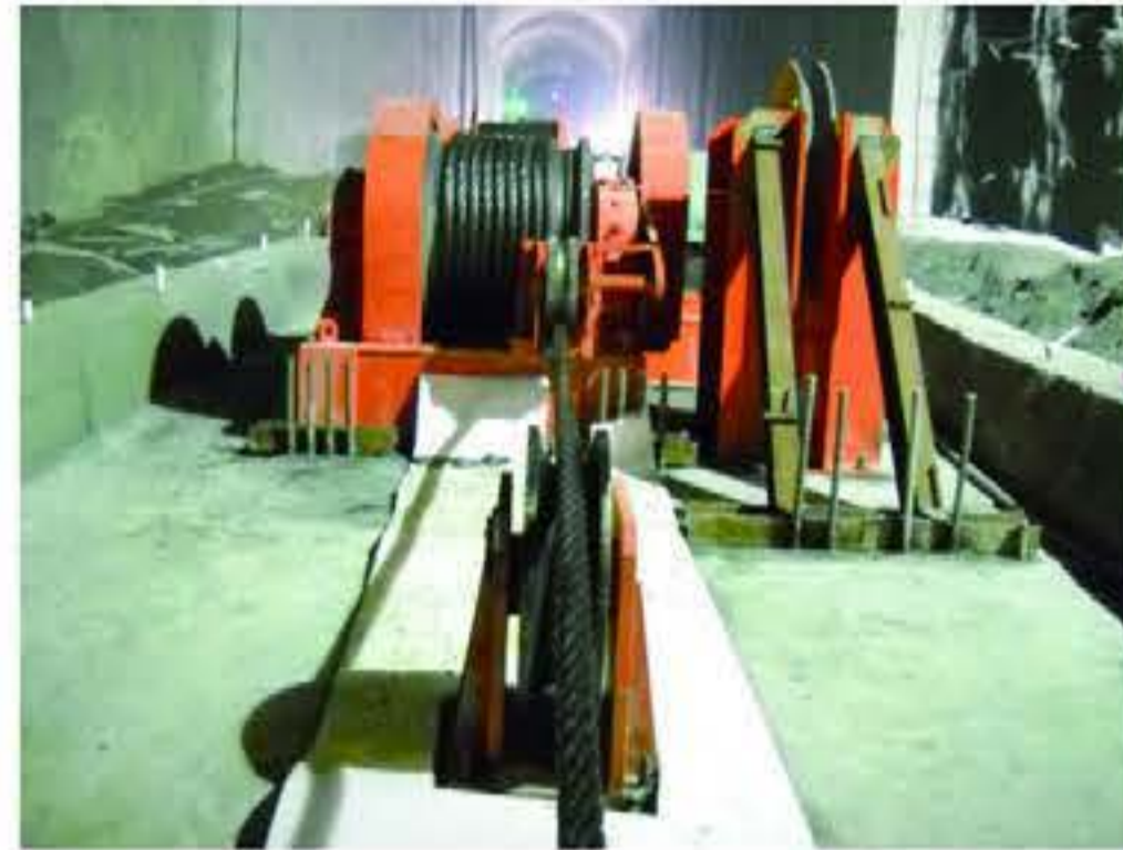
溪洛渡施工现场 xiluodu hydropower station
