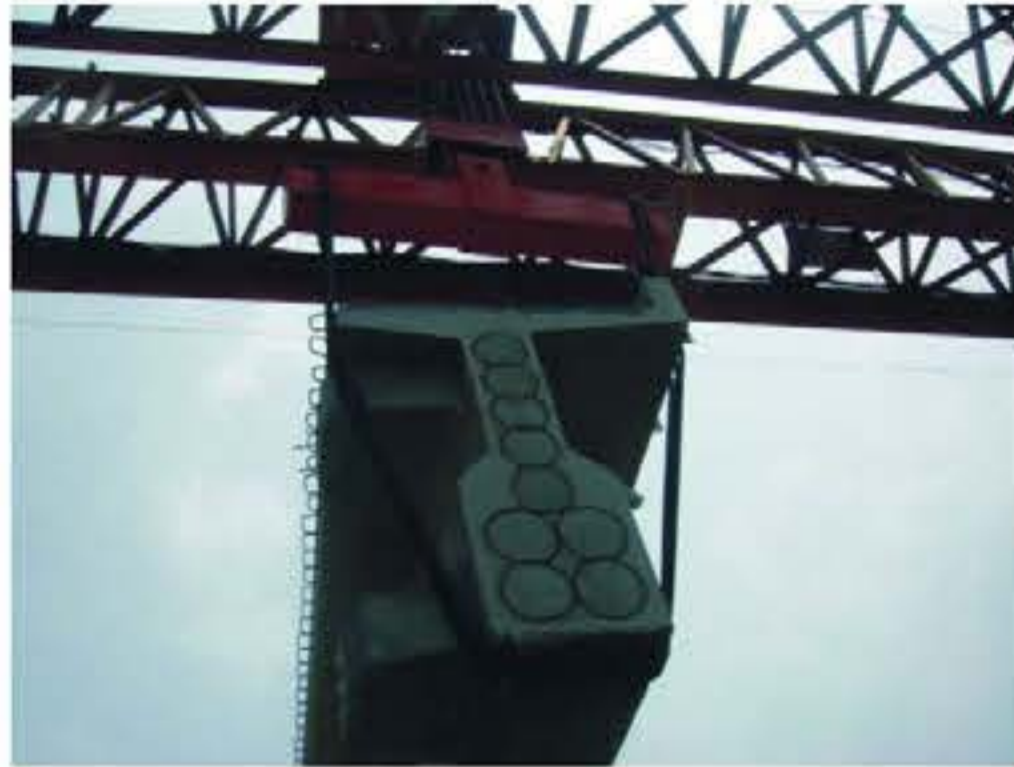
80t小车施工现场 80t winch trolley at site
