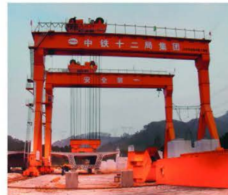
中铁十二局施工现场 China railway 12th group construction site
